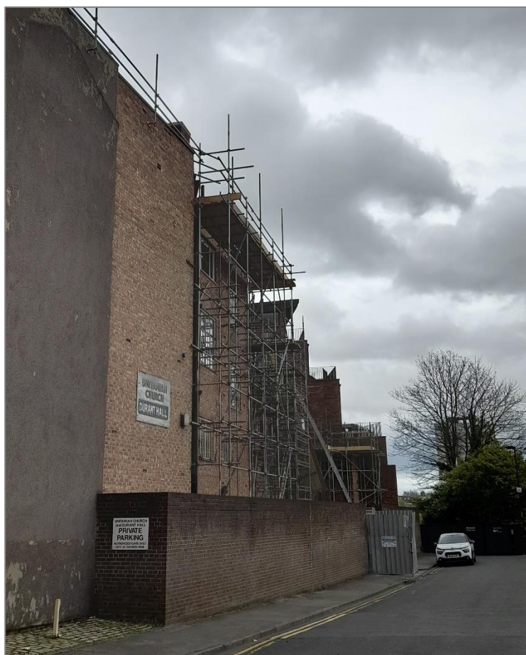
The start of work on our former building
